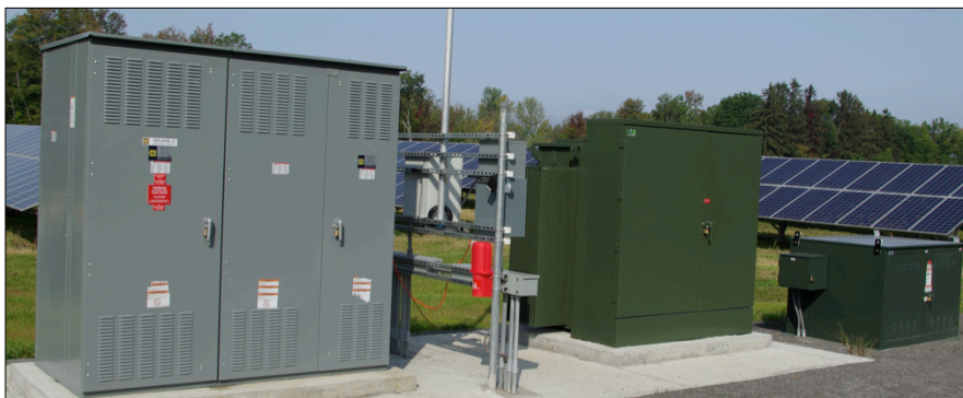
Pictured at left are the inverters changing direct current to alternating current
